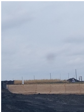
Jute Matting at MB-WC71-1054.200. Photo taken facing West
