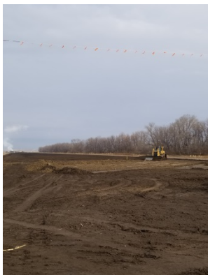
Dozer Pushing Dirt Rd.29, Photo taken facing North
